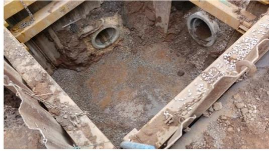
During the next 2 weeks the sheet pile capping beam up the A19 will be completed together with the combined 450mm dia combined sewer diversion.
